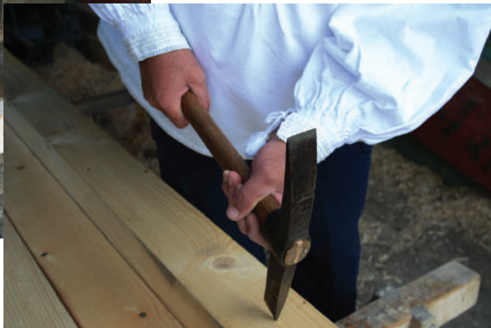
Ion Pop – Taina finishing a wooden beam using his wide-edged axe
