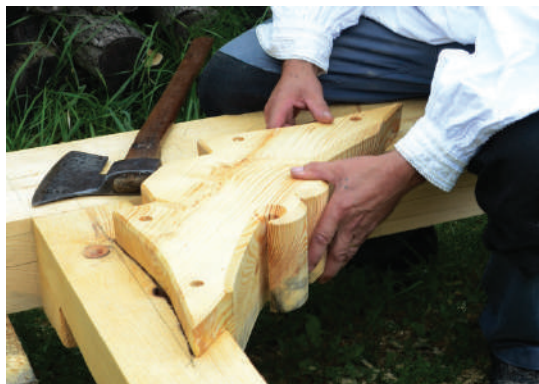
Vasile Pop carving “căpriori” (wooden poles supporting the porch roof) and “chitusi” (wooden bunch supporting the arcade of the porch)
